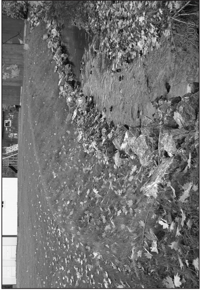
Laurel Run Creek project after reggrading, bank armoring and planting.
